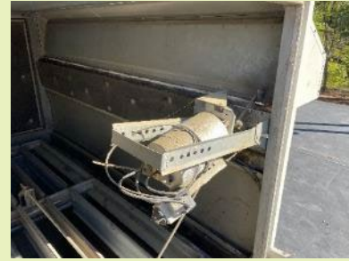
Maple Avenue Elementary Air Handler with Pneumatic Actuator
