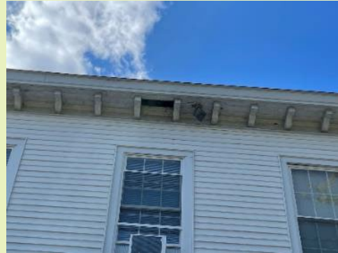
SAU Office Hole in Soffit
