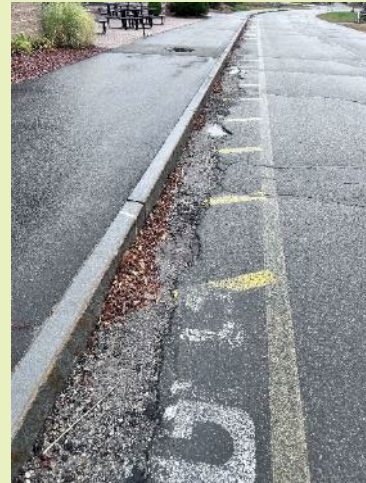
Goffstown High School Pavement Showing Signs of Deterioration
