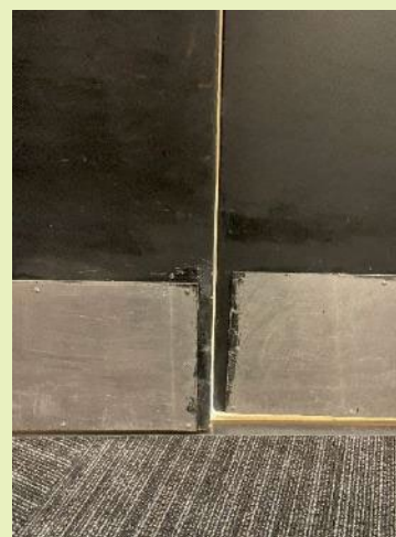
Goffstown High School Exterior Door Showing a Large Air Gap
